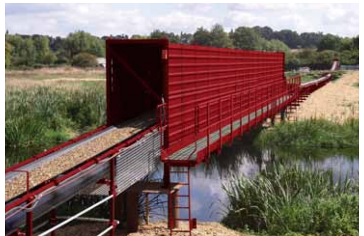
The conveyor passes from two access roads and crosses a river requiring a 25 m access bridge.
