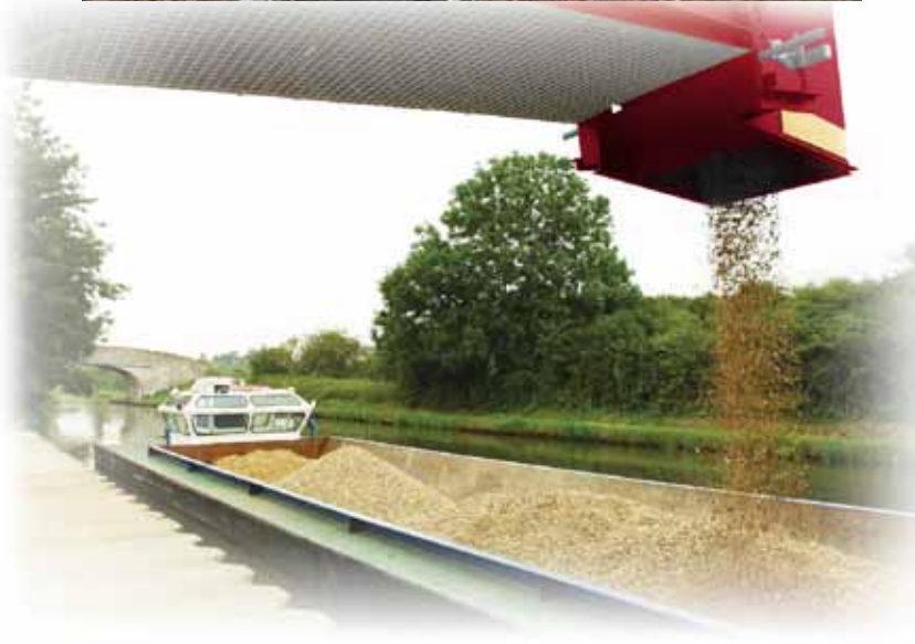
The complete conveying system was fully automated allowing for total control by the barge operator.
