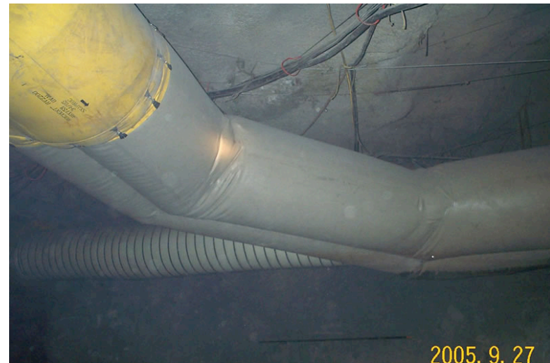
Engineered 90 degree, Duo Duct Elbox 8000ft. Level Kidd Creek
