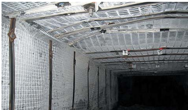
Tensar Mining Grids and UX Roof Mats provide effective rib and roof control for the most demanding applications.
