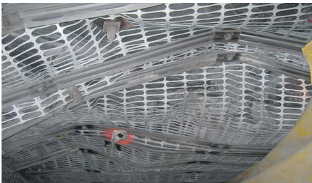
Tensor Roof Mats have greater surface area coverage which dramatically reduces the occurrence of rock fall through.
