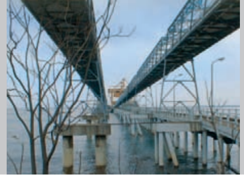
Harbor loading plant for coal and ore in Vado Ligure (Italy) with different conveyor speeds.
